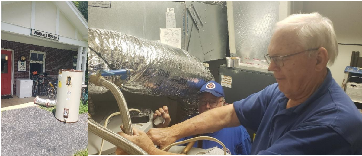
Ken & Klaus – Water Heater Install
