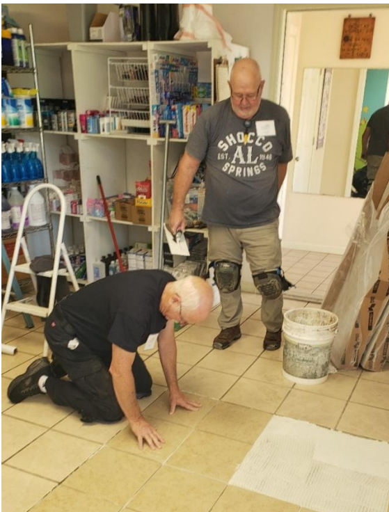
Jerry & Gary – Tile installation
