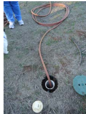
Pumping into a typical sewer cleanout port
